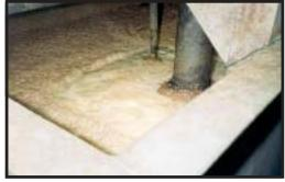
Sludge layer created by the aeration bubbles.
