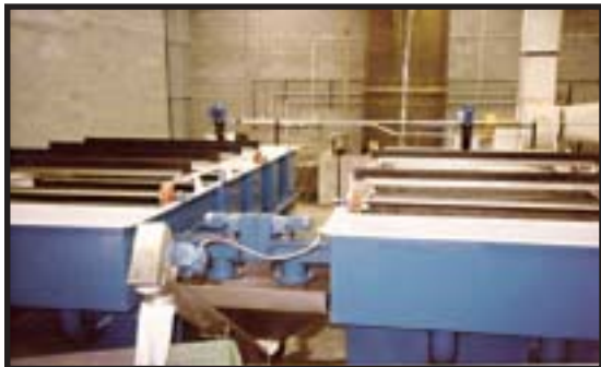
The two CAF-75 units operating side by side.
