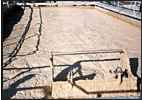
Sequential Batch Reactor (SBR) system.
