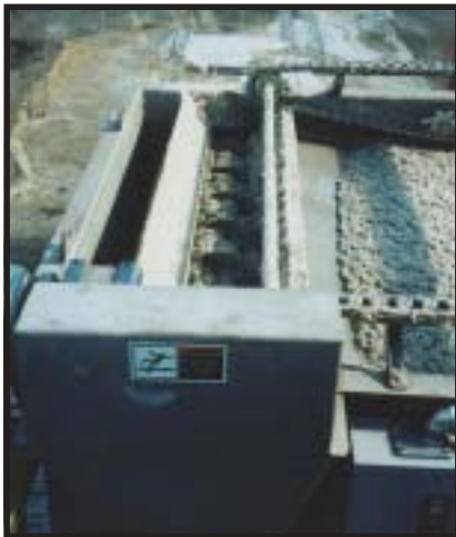
Sludge layer being scrapped into the auger chamber.
